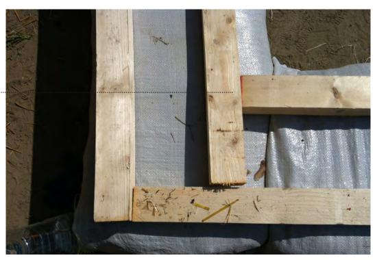
LINK THE BEAMS WITH METAL PLATES TO FORM A RIGID SYSTEM TO FIX THE STRAPS BELT AND CREATE THE BASEMENT FOR THE STRAW BALES
